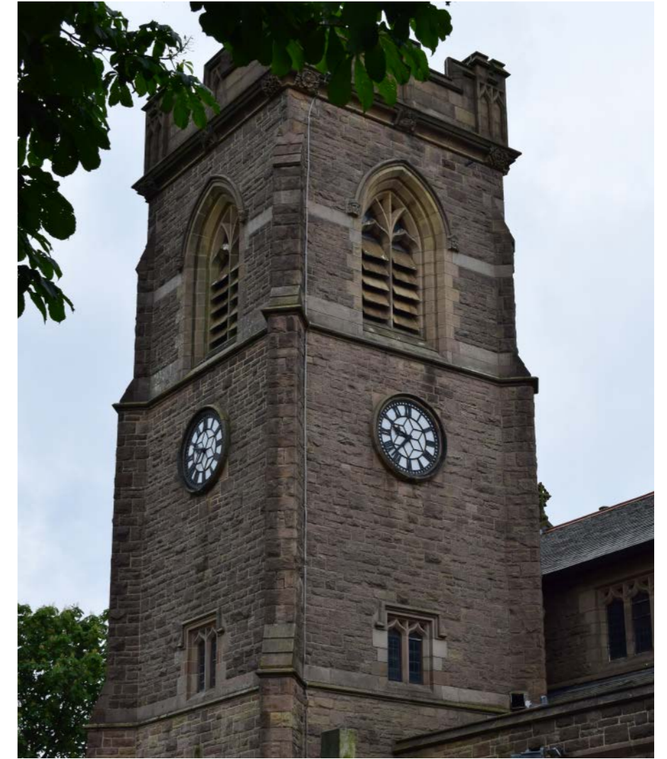
Image 4: St Johns Church and War Memorial, both of which are Grade II listed, sit to the south west of the site.
